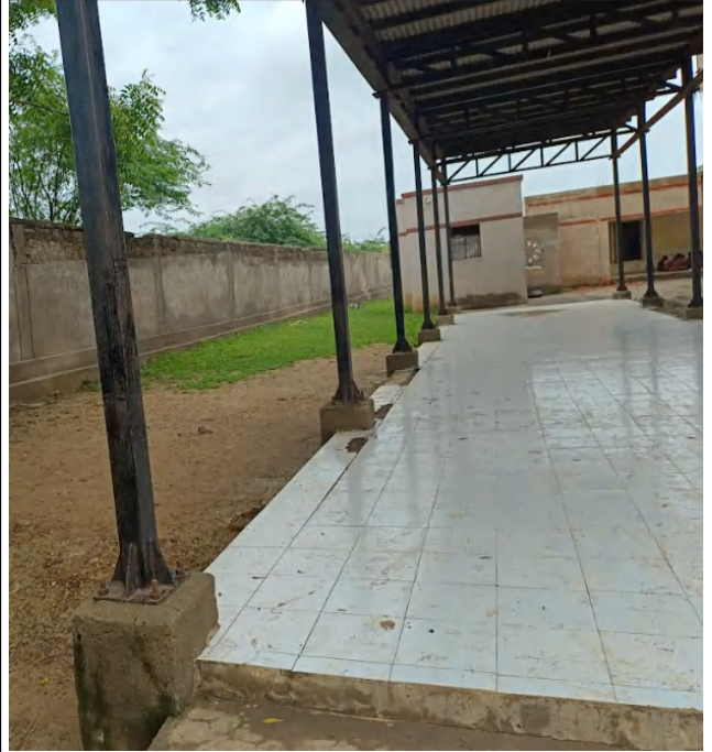
[Fig : Shed work and civil work at Junawad school]
