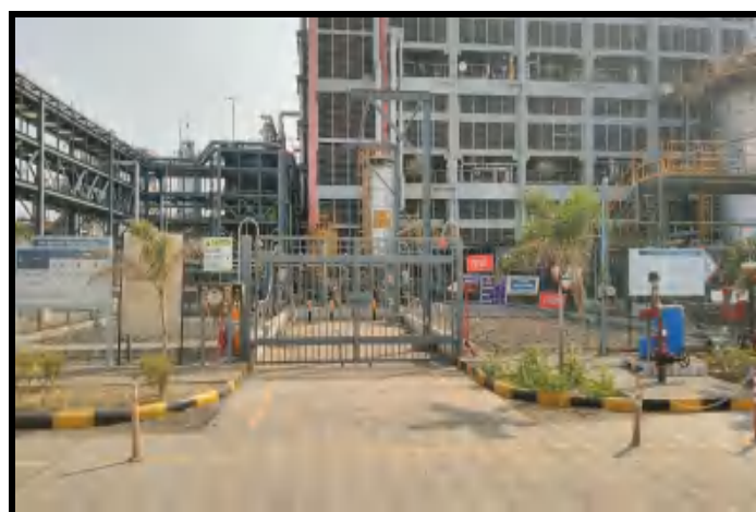
Photo of PESO tank farm area
