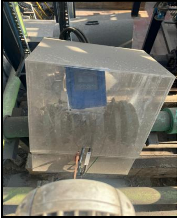
Flowmeter at NCT Discharge Point
