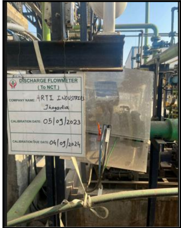
Flowmeter at NCT Discharge Point
