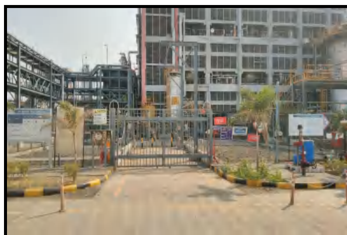
Photo of PESO tank farm area
