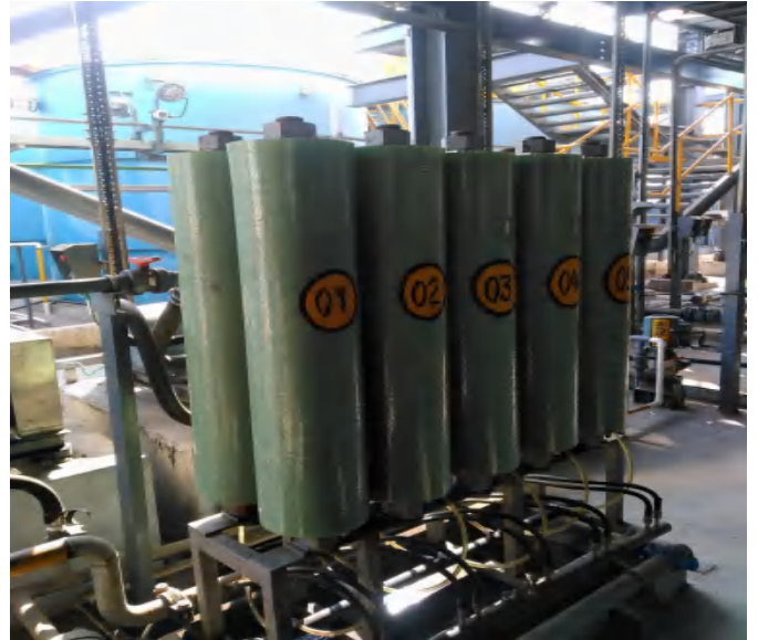
RO system capacity -135KLD
